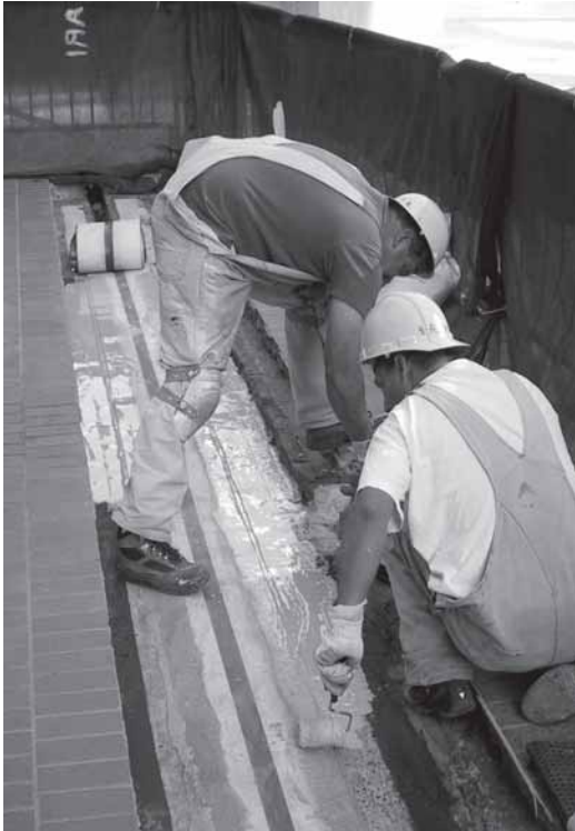
▲ Rolling in the liquid membrane on to the RedLINE.
