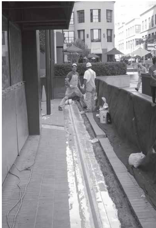
▼ The completed RedLINE expansion joint encapsulated in liquid membrane.
