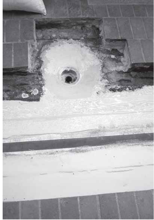
▲ A drain detail next to the RedLINE, note the liquid membrane continuity.
