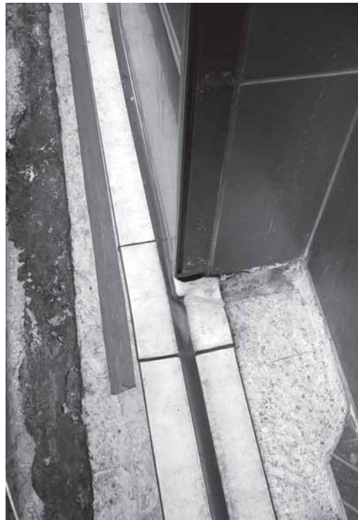
▼ RedLINE laid out at a detail on site prior to encapsulation.
